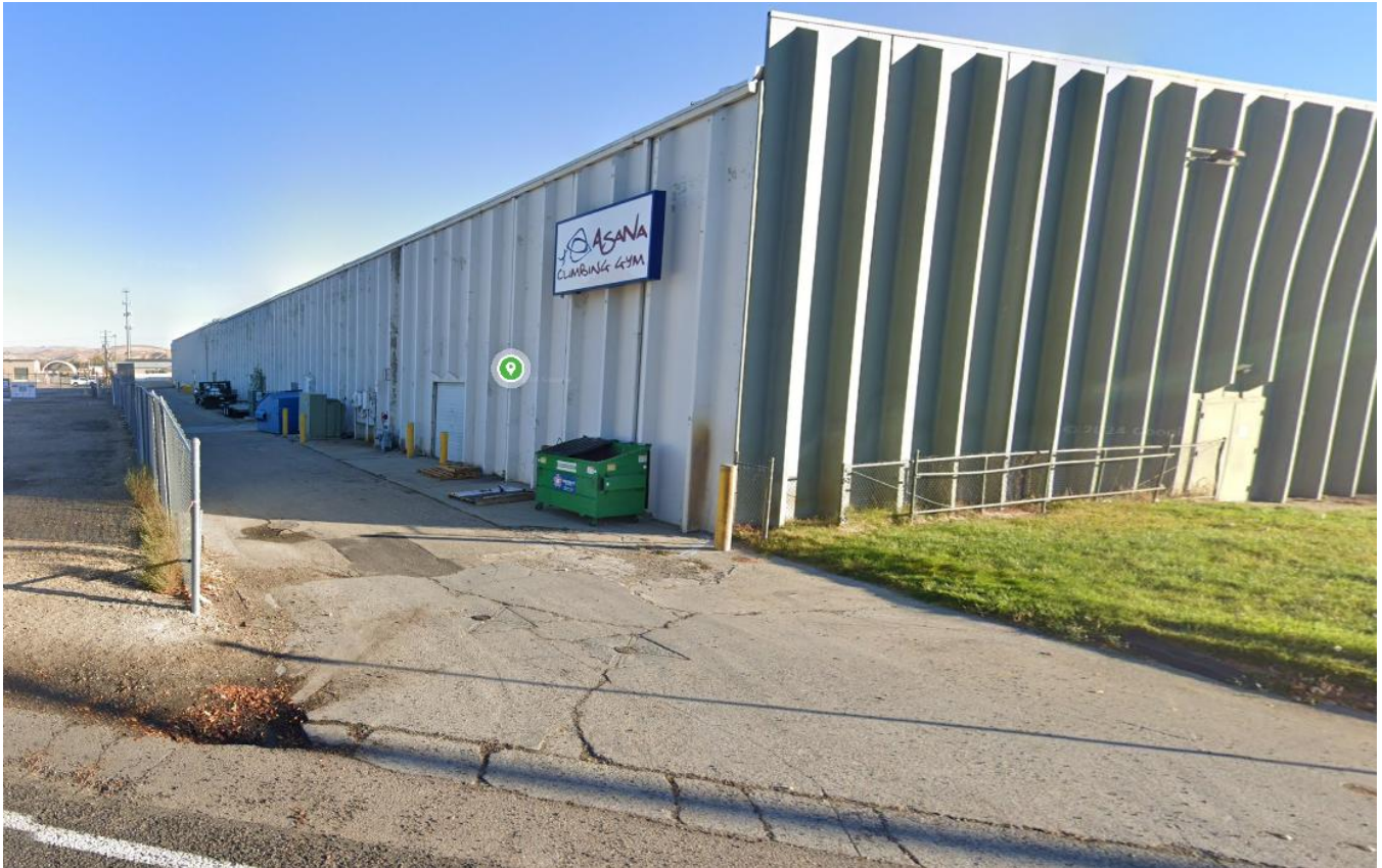
Figure 1. Dumpster location along Chinden Blvd.
